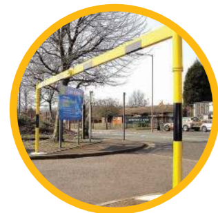
HEIGHT RESTRICTION BARRIER
